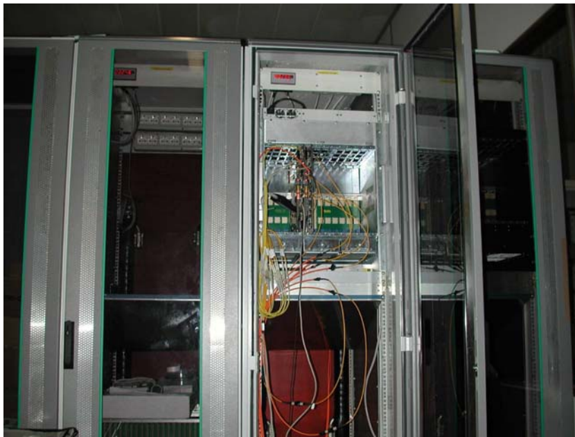
Figure 19.4: Racks for the pre-processing electronics, placed in the AGATA-PRISMA control room.
