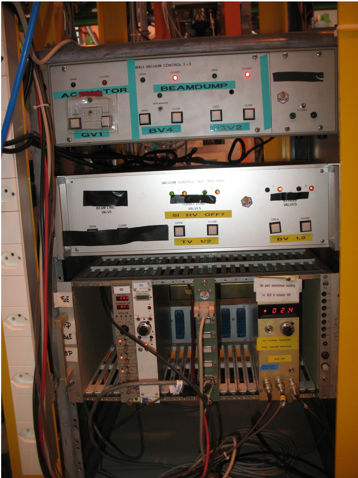
Figure 52: R6 (under beam dump): interlock and ionisation chamber
