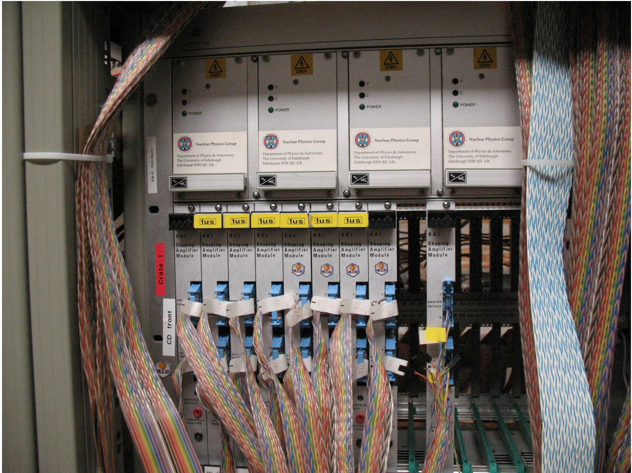
Figure 34: R2.C1: The RAL109s for the front rings. The upper connections are for the energy and they are joined up in pairs and sent to the ADC. The lower connections are for the timing and they go to the MALU in R1.C2 and from there to the TDCs in R3.C1.
