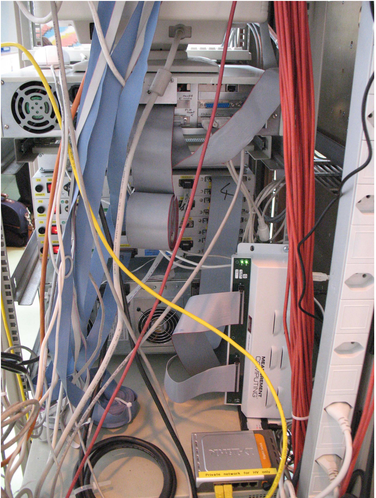
Figure 55: R5 rear: autofill connectors
